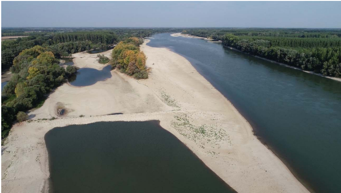
Figure 33 Side arm sedimentation near Vének at rkm 1798 rkm (source: ÉDUVIZIG, 2018)
