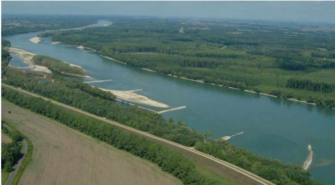
Figure 26 River engineering structures at low level around rkm 1799 (aerial photo taken in 2011)
