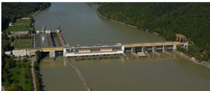
Figure 21 Hydropower plant Aschach at the Danube River (photo: Verbund AG)
