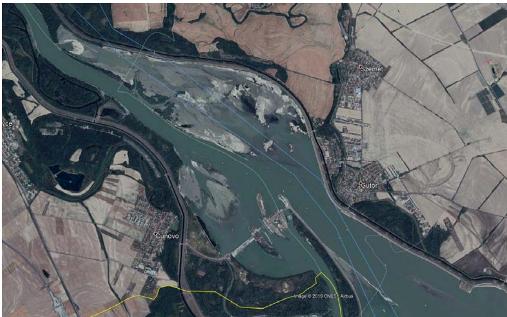
Figure 41 Sediment deposition zones upstream of Gabčíkovo dam (Google Earth).
