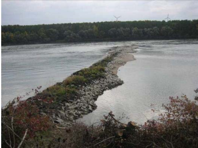
Figure 14 Orthogonal groyne at mean water level (as a consequence of river bed degradation) (Habersack et al., 2012)
